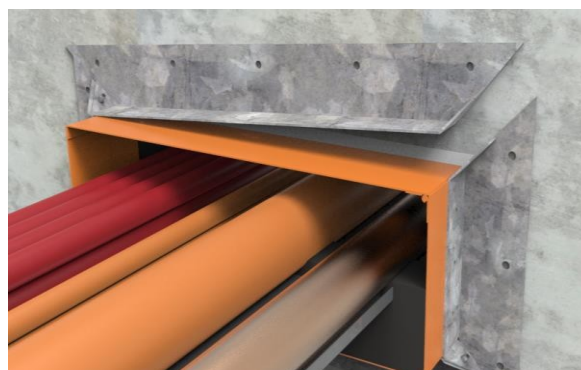
Fit the flange over around the box
